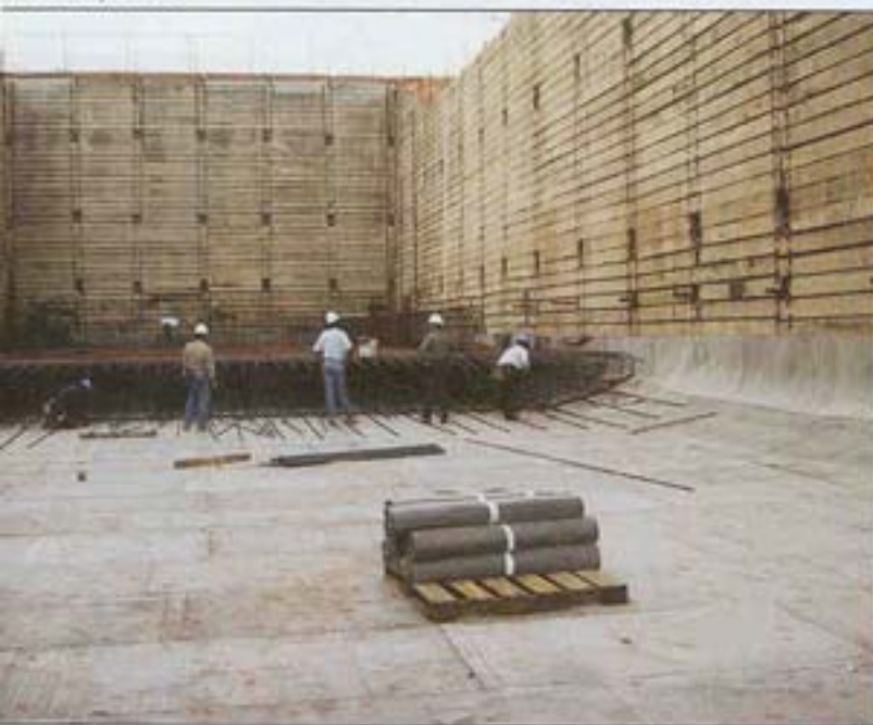
A look at the slab edge of the tunnel construction project at George Bush Intercontinental Airport.
