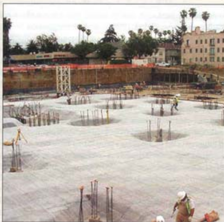
(Above) When hydrated, bentonite expands and conforms to penetrations and irregular surfaces, sealing small concrete cracks. (Right) Bentonite systems can be installed directly onto compacted soil or gravel substrate without a working mud slab.
